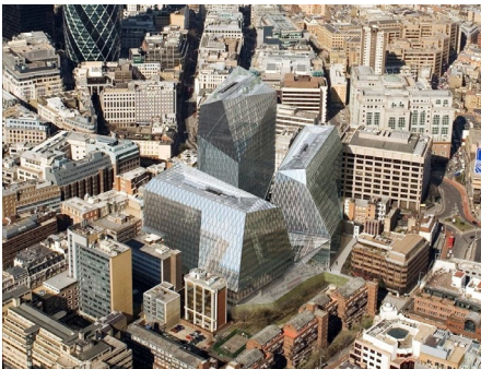
TRINITY EC3 OFFICE COMPLEX London, UK
