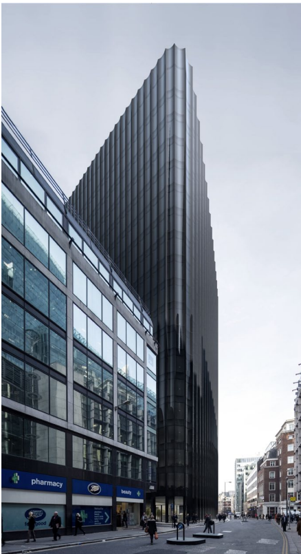
130 FENCHURCH STREET City of London, London, UK Completion date: 2020
