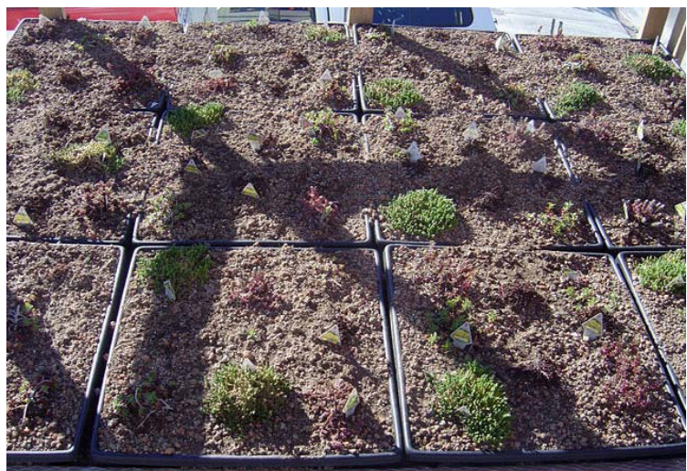
Photo of test roof on construction trailer
