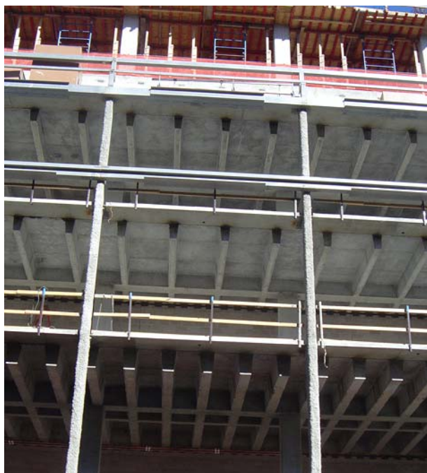
Construction photo of structural system
