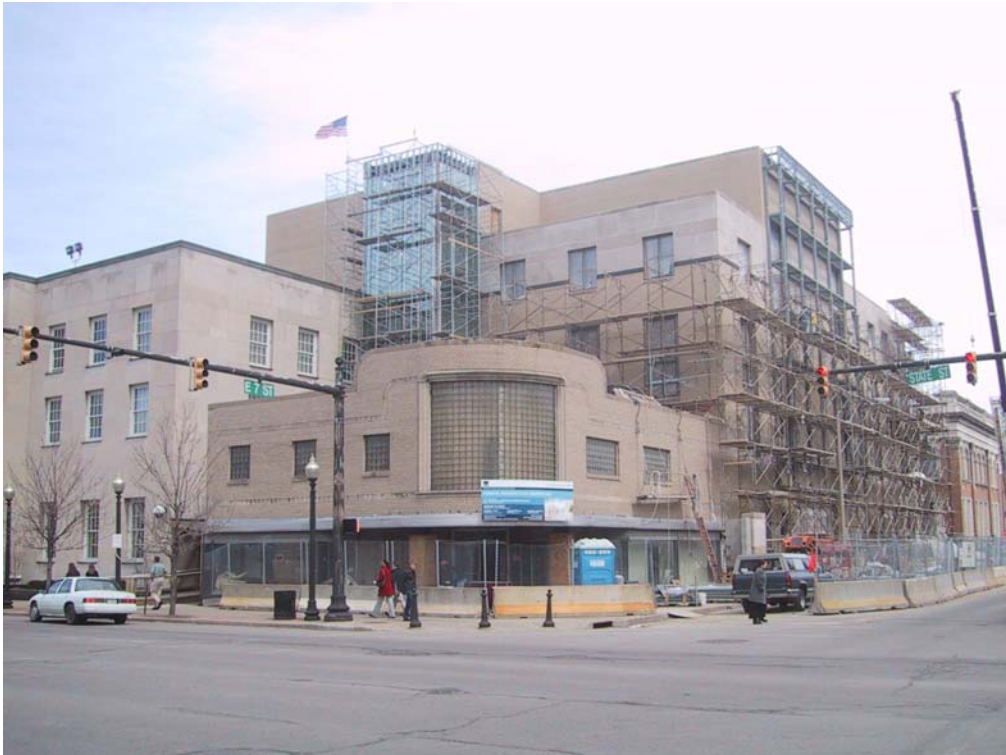
Figure 5: Annex under construction in April 2003 (photo by author)
