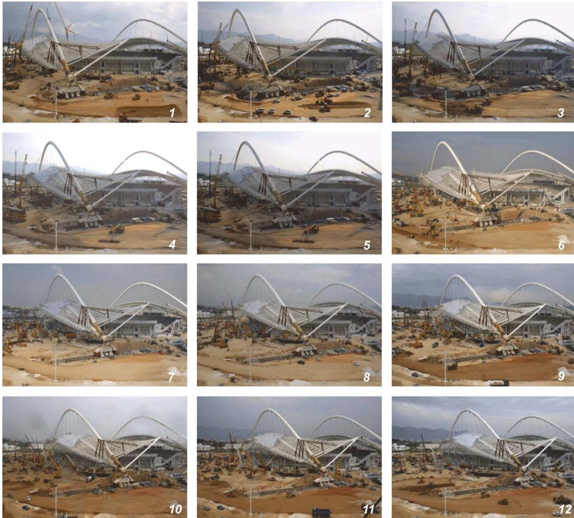
Fig. 17. Sliding sequence of the east arch.
