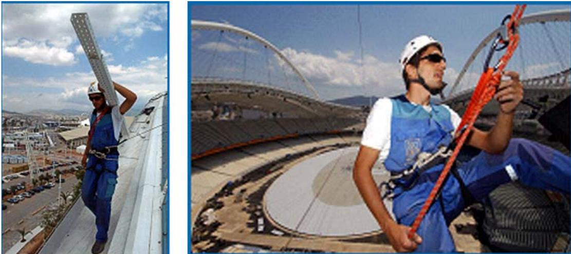
**Fig. 20.** Steel wires and safety belts protect the workers when working on top of the arches.
