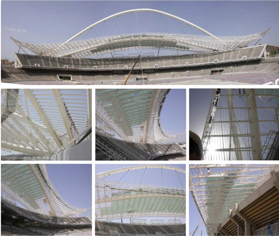
**Fig. 18.** Installation of girders, perlines, and polycarbonates.
