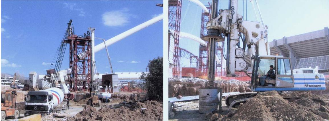
**Fig. 10.** Excavation and foundation of the support piers.
