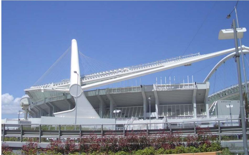
**Fig. 24.** The completed stadium of OACA, showing the torsion pipe and the arch on the west side of the stadium.
