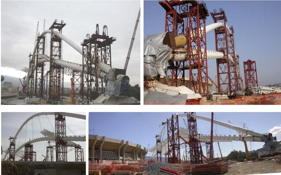
**Fig. 12.** Steel pylons supporting the structure. Suspension with steel wires and installation of girders.
