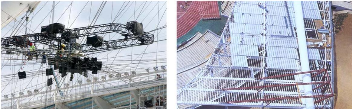
**Fig. 21.** Spider web and installation of M&E along with the placement of the polycarbonate panels.
