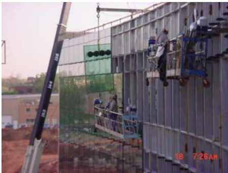
Curtain wall assembled on robust structural frame.
