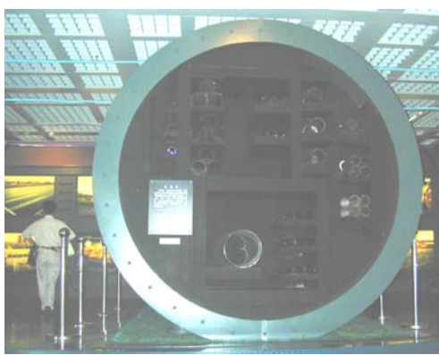
Fig. 17: A large conduit for carrying the city's services in an organized way (Shanghai City Museum).
